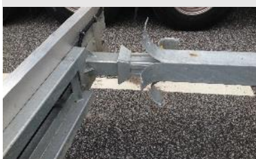
Damage by crash with about 35 km/h
